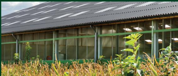
The insulated build up commonly used for poultry housing is ideal to achieve this and when used in conjunction with Eternit sheeting the building will have excellent thermal and acoustic performance along with the longevity expected to exceed the service life of the unit.
